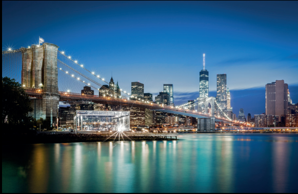
Drinking Water Network Monitoring for Smart Cities
